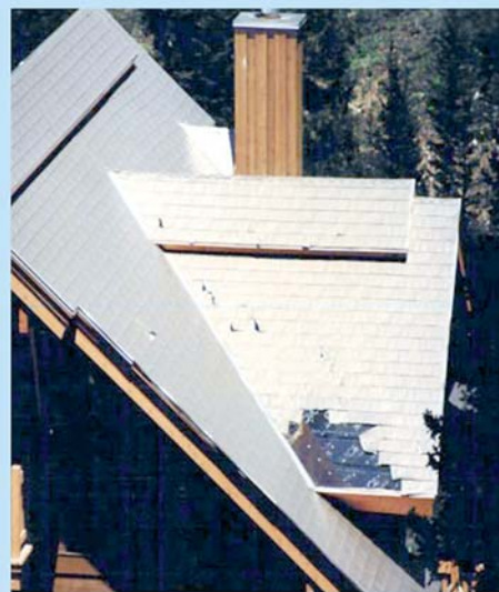
Photo 1: Damage to flat seam metal roofing.
